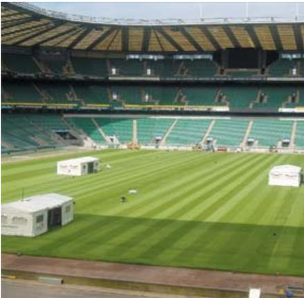
The old pitch consisted of four inches of fibre sand with five metre drains laid on the original cabbage patch. It served the game remarkably well but was ageing and the drainage slowing, sometimes leaving standing rainwater. Now, whereas the old drainage allowed 20/25mm of water to drain away in an hour, the new one copes with between 150mm and 250mm.
